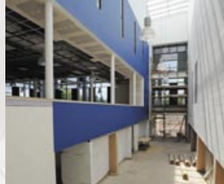
Bearden Academy, Glasgow while under construction
